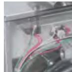
**Reliable** Direct hot surface ignition system features an advanced silicon nitride igniter and in-shot burners for greater reliability.
